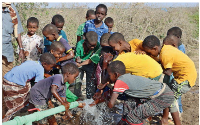
The new boreholes we drill and the new wells we dig bring safe water to hundreds of thousands of people across Somalia each year
