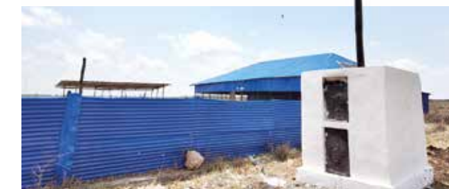
Rehabilitating health centres, like this one, to deliver health services was an important part of the SHIP and MSER integrated projects
